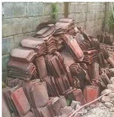
Figure 1. Used roof tiles piled up around the house (Photo: Marwanto 2021)
