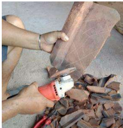
Figure 4. Cutting used roof tiles using a grinding machine (Photo: Marwanto 2021)
