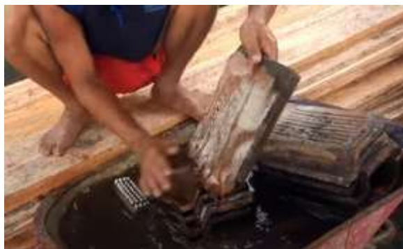
Figure 2. Washing used roof tile to remove dirt and fungus (Photo: Marwanto, 2021)
