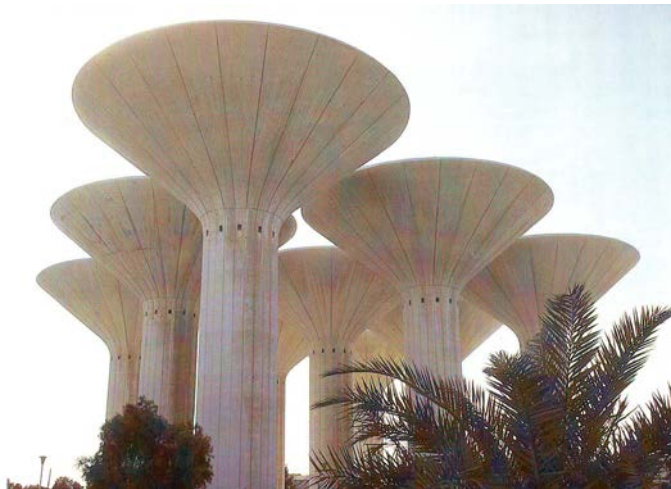
Kuwait Water Tower (1978), Lindstrom, Egnell & Bjorn. Sumber : Introduction to Architecture, 1993.
