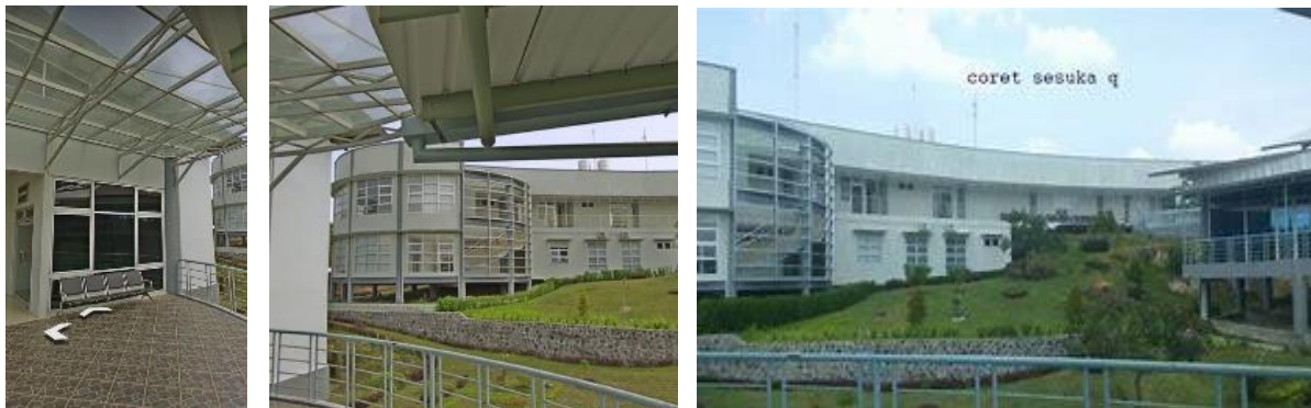
Fig. 2. Modern Design of Buildings
