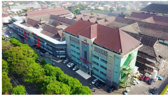
Fig. 1. Aerial view of Dr. Moewardi Regional Hospital. Source: rsmoewardi.com
